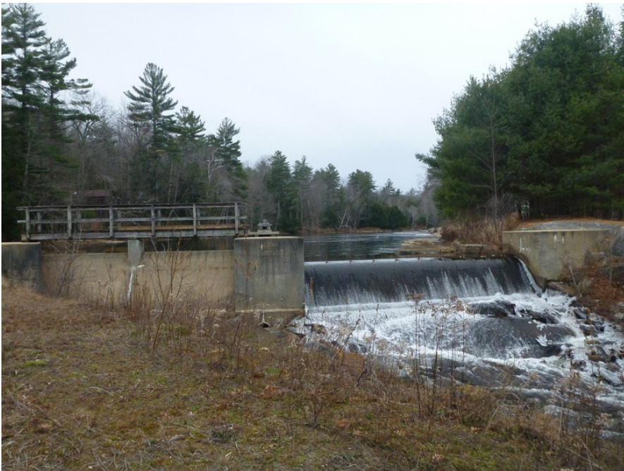
Figure 8.1. Gregg Lake dam, rebuilt in 1982, with no flashboards in place.
