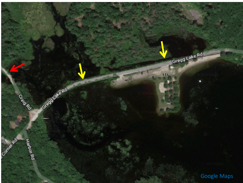
Figure 5.7. Overhead view of the causeway stretch of Gregg Lake Road, including the Town Beach and Boat Launch area. Arrows show locations of sinkholes that opened up along Gregg Lake Road (yellow) and Craig Road (red) in 2018.
