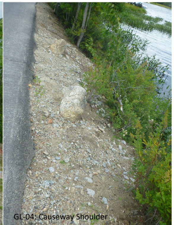
Figure 5.9. Erosion Sites 03 and 04, showing bare shoulders and erosion of steep banks leading directly into Gregg Lake.
