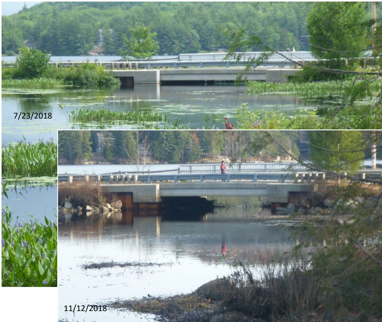
Figure 5.10. The Gregg Lake Road bridge with the water on the north side of the beaver dam nearly touching the bottom of the bridge in Summer 2018, and in Fall 2018, following removal of the beaver dam.
