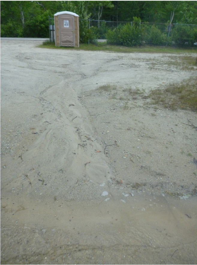
Figure 5.14. Stormwater flow down the public boat ramp into Gregg Lake.
