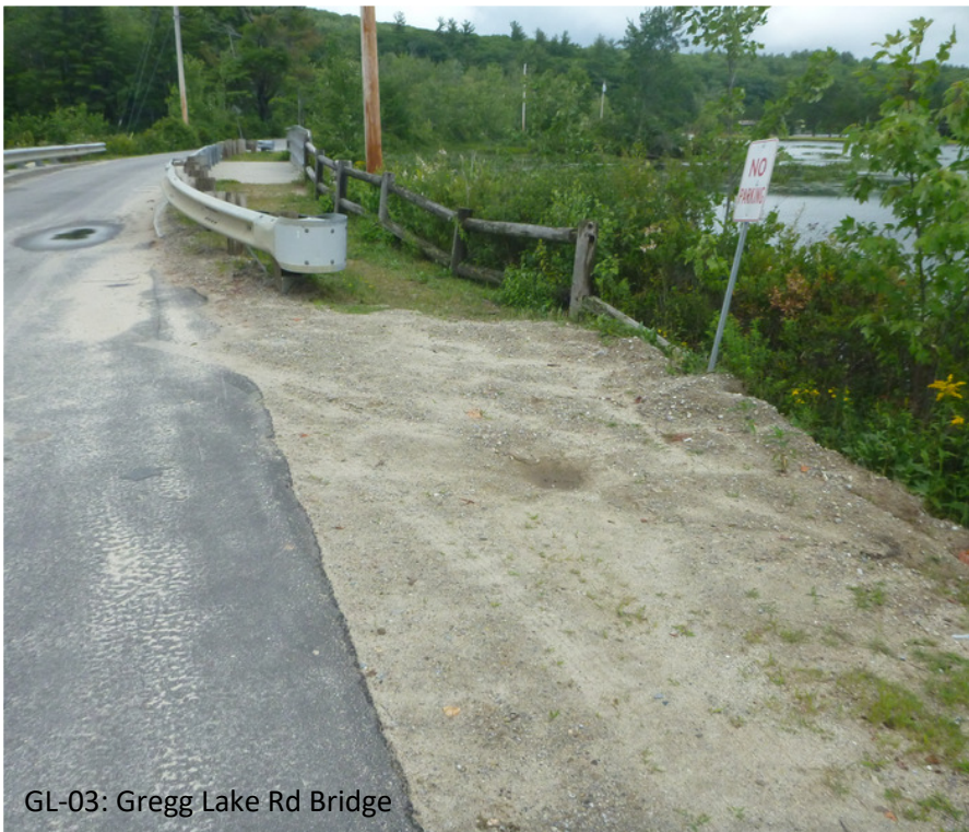
Figure 5.9. Erosion Sites 03 and 04, showing bare shoulders and erosion of steep banks leading directly into Gregg Lake.
