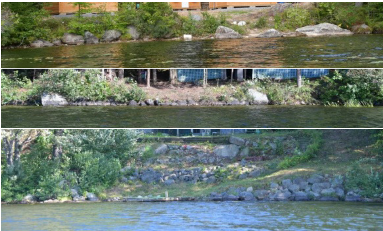
Figure 6.2. Examples of recent clearing, exposing shoreline to erosion at Gregg Lake.
