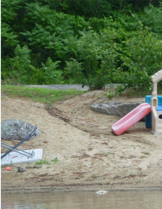
Figure 6.4. Erosion Site 11, where runoff from Holt Hill Road flows across a private beach, carrying phosphorus and sediment into Gregg Lake.
