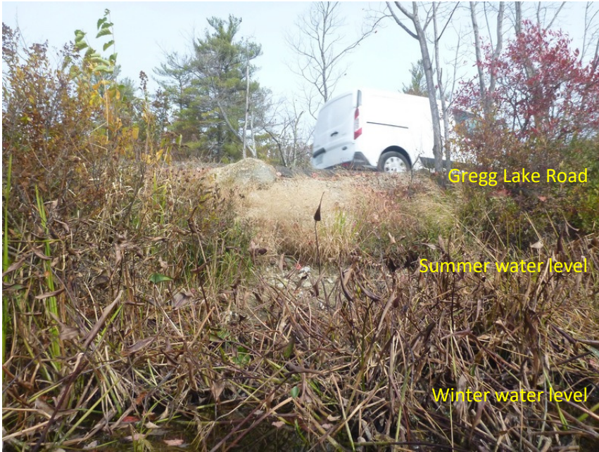
Figure 5.8. Loss of vegetation and erosion at steep causeway bank, visible at winter water level.
