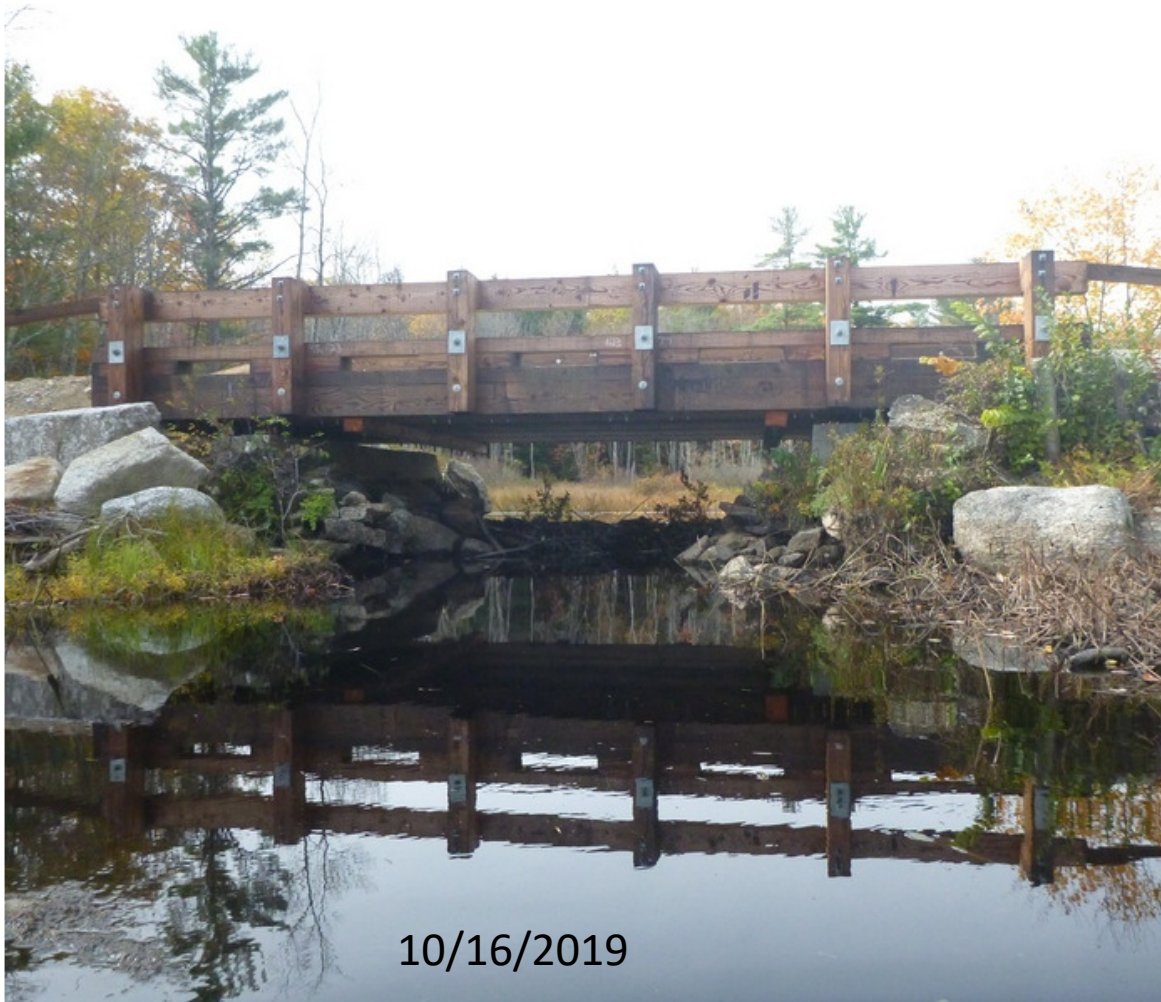
GL-06: Craig Road Bridge
