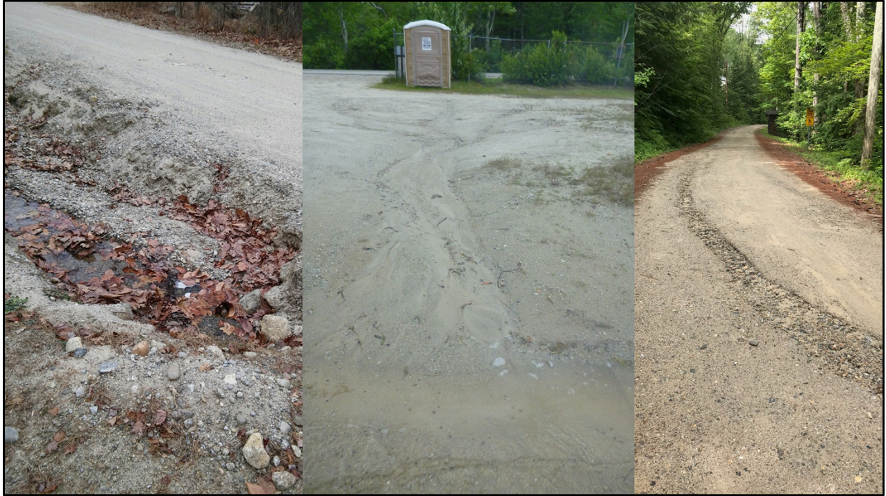
Road erosion issues, bank stability, lack of buffers, sediment carries phosphorus into the lake and river
